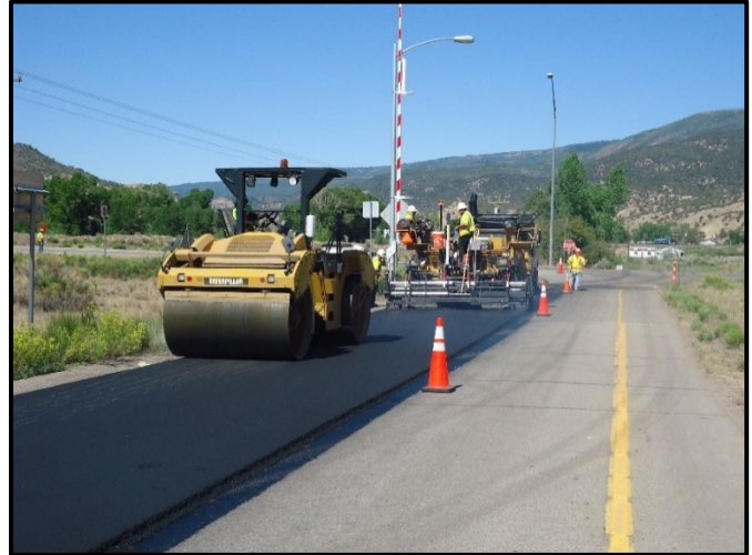
Roadway asphalt paving operations
