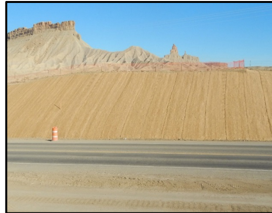
Soil Retention Blanket application on slopes
