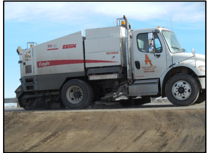
Sweeping and Vacuuming operations
