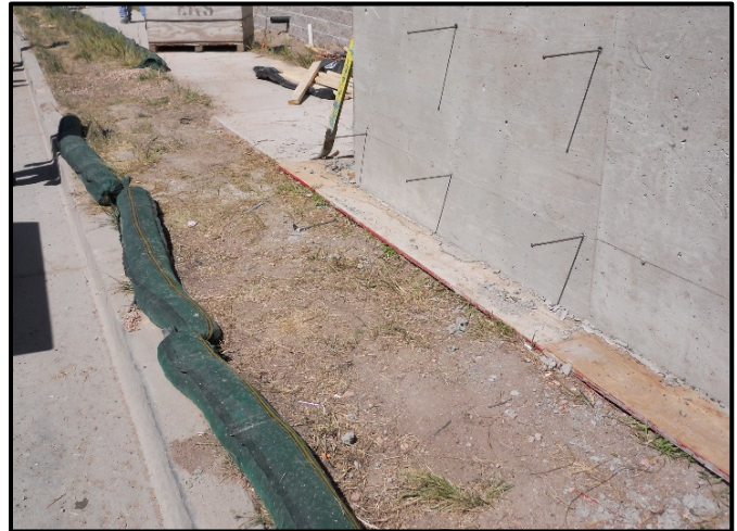
Aggregate Bag used for temporary sediment control
