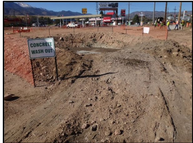
Concrete washout structure
