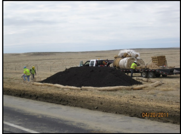
Erosion Logs used for stockpile management practices
