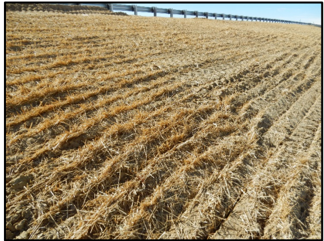
Straw Mulching on disturbed side slope
