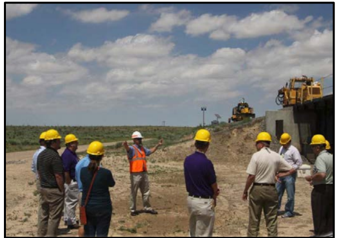
On site work coordination
