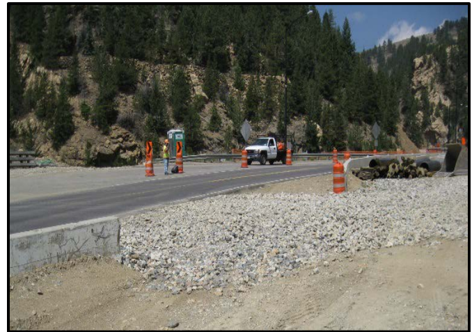
Vehicle tracking pad at entrance of construction site
