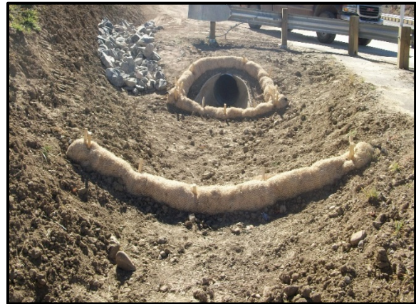
Erosion Logs along construction access road
