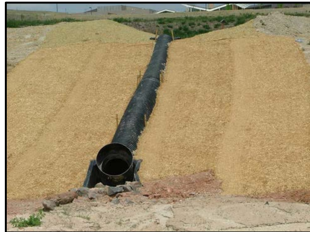
Temporary Slope Drain on stabilized slope
