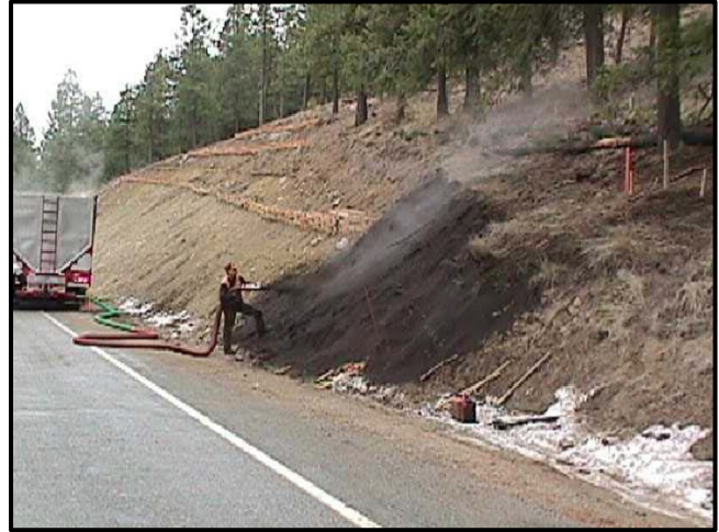
Compost Blanket Applications on Slope
