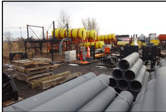
Site Waste and Materials Management
